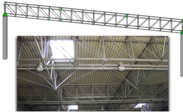
Fig. 6 – Main truss view.
