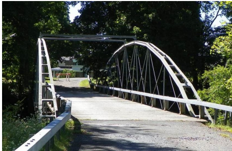
Fig. 2 – Whipple Bowstring Arch bridge, S. DeGraff (Syracuse, NY) 1867-'69 ( https://upload.wikimedia.org )
