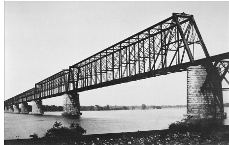
Fig. 3 – Cairo Bridge's 2 157.9 m built by Whipple's plans ( https://upload.wikimedia.org )
